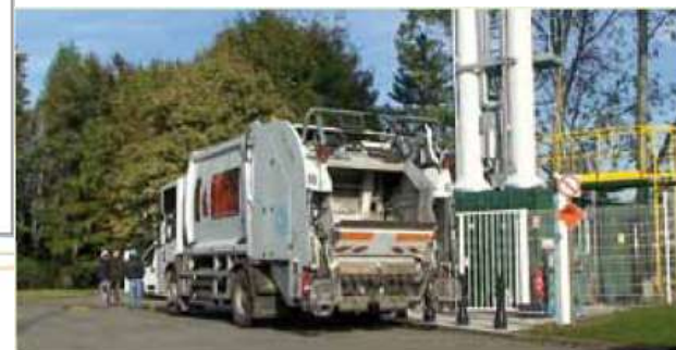
Trucks refuelled at the upgrading plant
